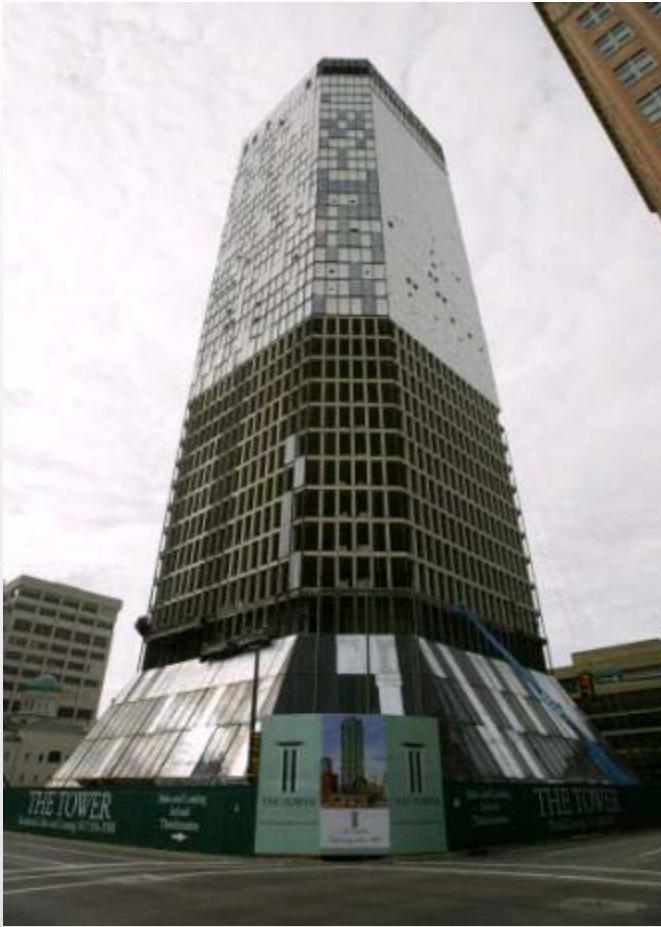
OLD FAÇADE - OFFICE BLDG
